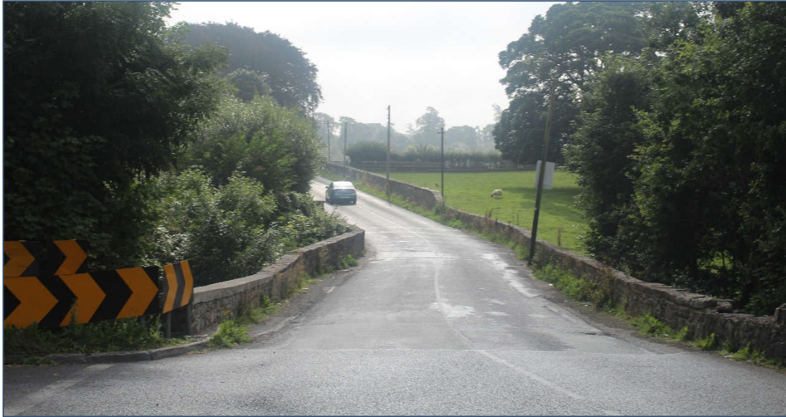
Plate 11-11 Bridge over the Blackhall Little on the L2214-3
