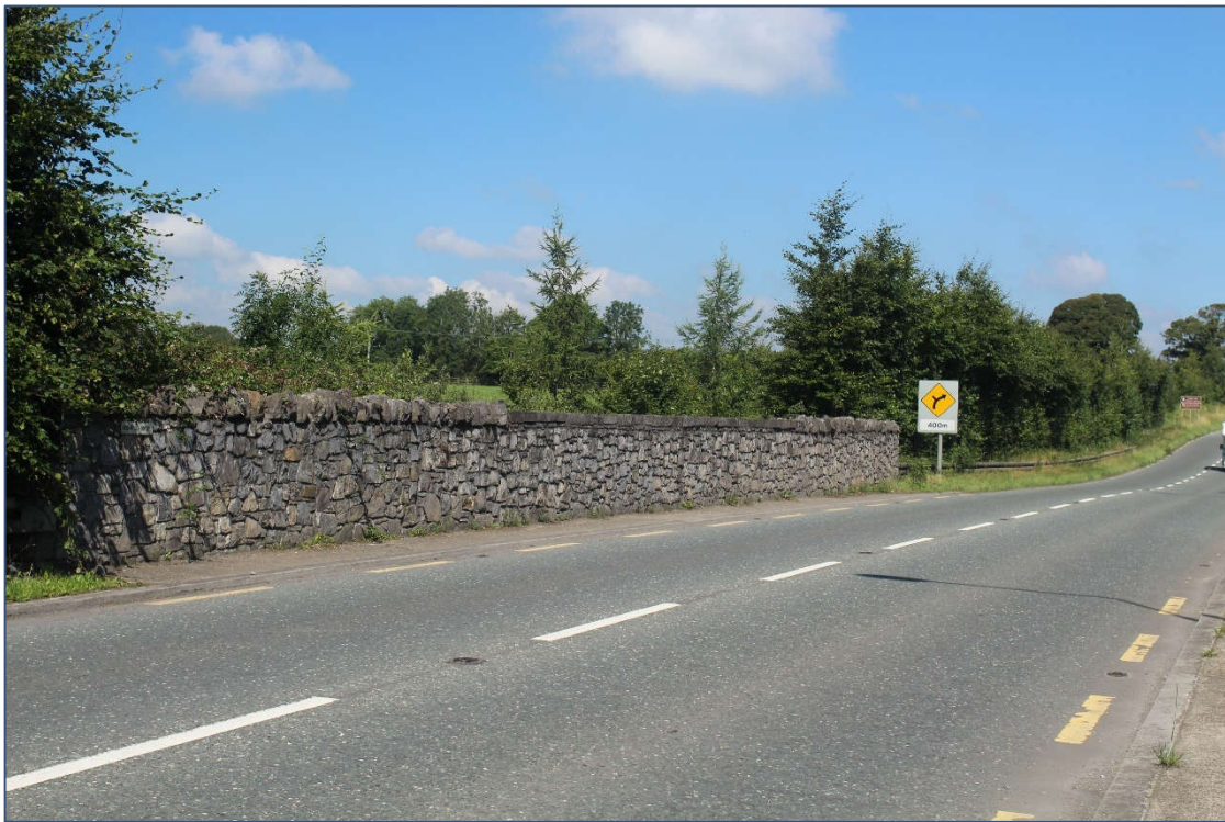
Plate 11-37 View north-east towards the Proposed Development from Kildare Bridge, on the R157 Regional Road.
