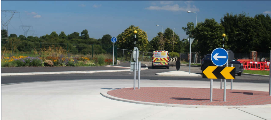
Plate 11-28 A roundabout on Moyglare Hall Road, where the proposed MOOR and Moyglare Bridge will link the Existing Road Network in County Kildare
