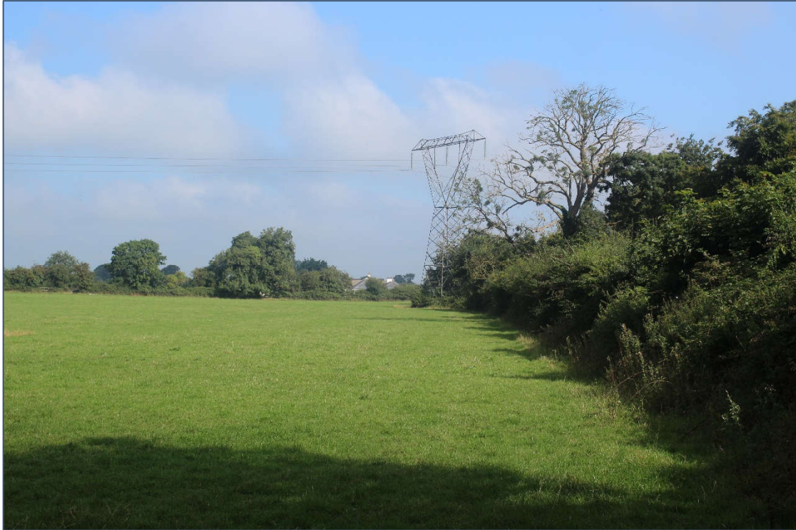
Plate 11-8 An electricity pylon at the north-east of the site where the MOOR will cross this field, parallel to the overhead line. Residential settlements are seen beyond the northern margin of the site boundary.
